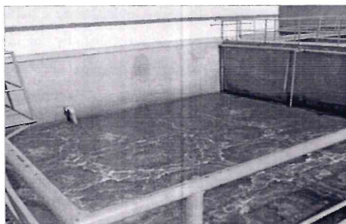
Figure 7 Equalization Tank
