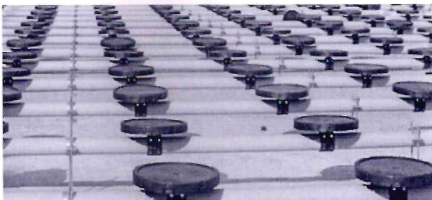
Figure 8 Course Air Bubble Diffusers
